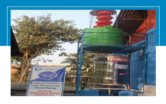
Installing a simple traditional hand pump for the provision of raw water. Keeping in view the ground situation, Bio Sand Filtration is added, an open aeration & electrical pump makes it a productive project. Filters water from turbidity (sand, silt, & clay); color; taste; and smell; providing 500 liters/hour.
