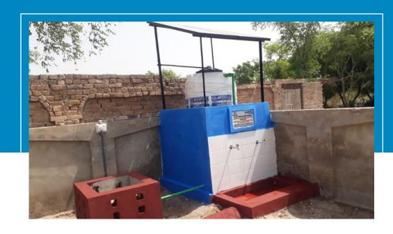
Installation of smaller size submersible pump, which is solar powered to lift water into a 500 liters water storage tank. Water for drinking and other use is taken via taps installed on two sides of the project.
