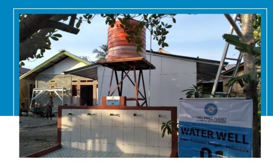
Boring underground 100+ feet to get water, which is pumped into water tank to be used through taps. Life of project is 3+ years; & with some maintenance, life of the project is further enhanced on periodic basis.
