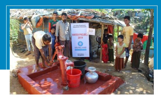
Dig deep underground around 1,000 feet to fetch water, which is taken out using hand pump. Life of project is 3+ years; & with some maintenance, life of the project is further enhanced on periodic basis.
